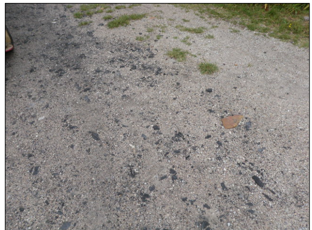
Gravel/coal surface cover of driveway
