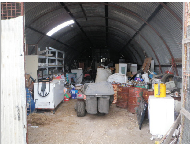
Inside shed igloo (BH30-20)
